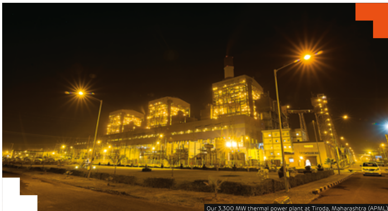
Our 3,300 MW thermal power plant at Tiroda, Maharashtra (APML)
